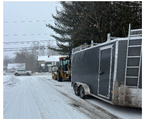
Water Main Repair in Gardiner
