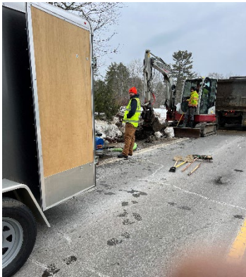
Water Main Repair in Damariscotta
