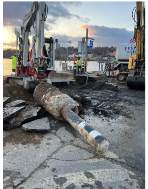
Sewer Force Main Repair at a Pump Station in Damariscotta
