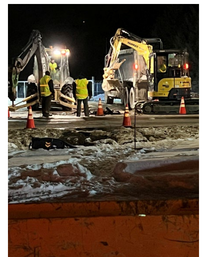
Water Main Repair in Gardiner
