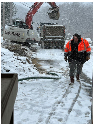
Water Main Repair, Solon
